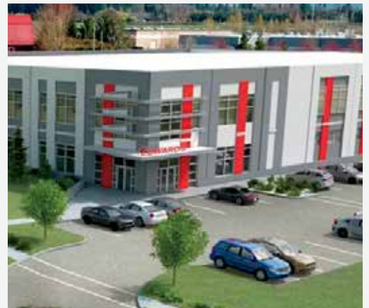
State-Of-The-Art 5,000 Sqft Facility
