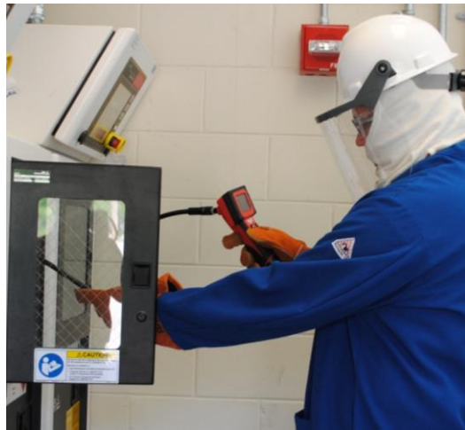
Fig. 22: Fiberoptic Scope Inspection
