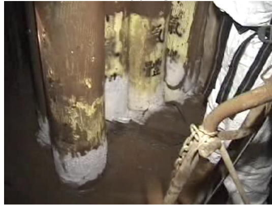
Fig 8: Removing ammonia cylinders frozen to ground
