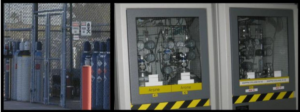
Figure 4 – Left: Metal hydride cylinders in storage yard before transport.
