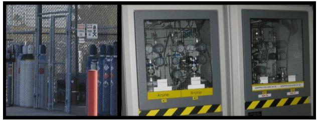
Figure 4 – Left: Metal hydride cylinders in storage yard before transport. Right: Arsine and silane 49 L cylinders in gas cabinets in a GaAs manufacturing facility.
